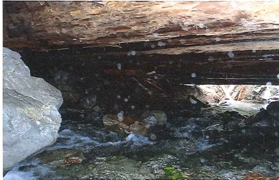
CK2066 Left Abutment
