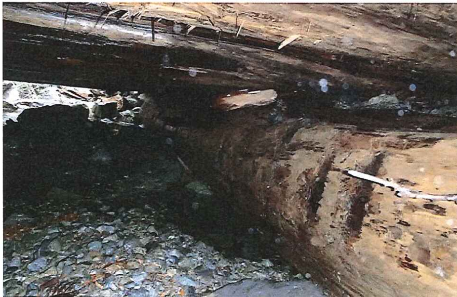
CK2066 Right Abutment
